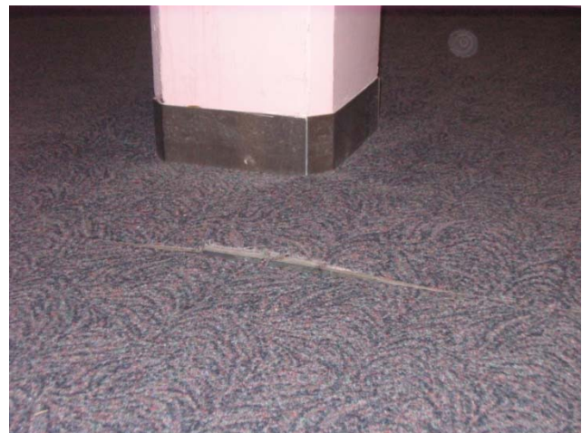
Figure 7: Carpet peeling up in 1992 Wing
