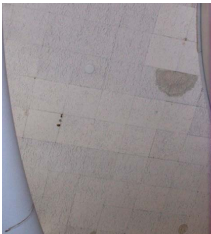
Figure 9: Water-stained ceiling tiles, 1992 Wing
