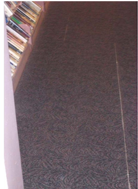
Figure 5: Carpet peeling up in 1992 Wing
