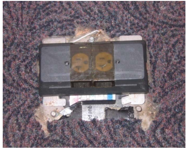
Figure 8: 'Tombstone' electrical receptacle in the 1992 Wing
