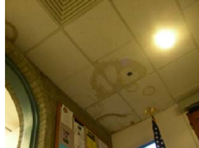
Figure 20: Water marks on acoustic ceiling
